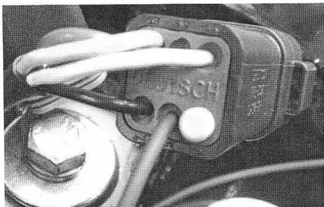
Figure 9—Finished Main Harness Connector
